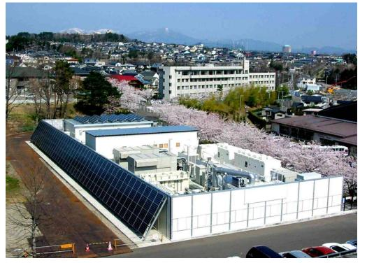
Great East Japan Earthquake (2011): Power was supplied to important loads by microgrid (Utility grid: blackout for 3 days) Source: NTT
