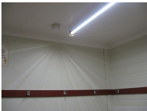
Figure 6 Beam distribution of un-diffused clear LED tube shows up on the squash courts change room wall
