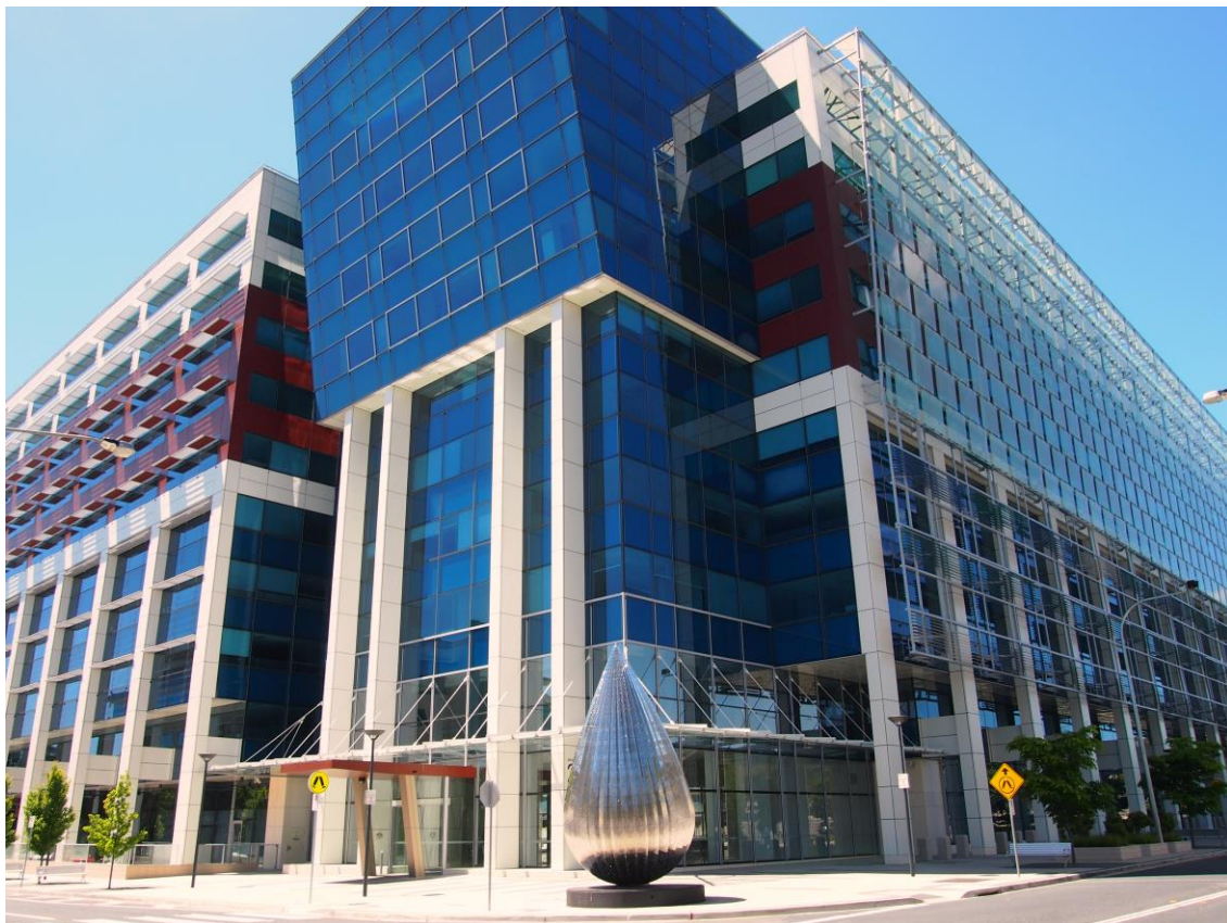
Figure 8. Sirius Building, Canberra. The shaded western façade is visible to the right; lighter shading on the northern façade is visible to the left.
