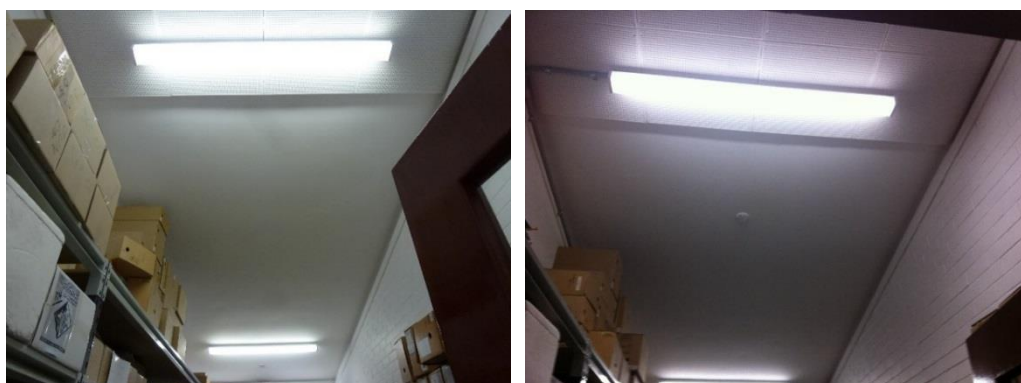
Figure 5 Suburban Community Hub #1 archive room fluorescent battens before (left) and after (right) upgrade
