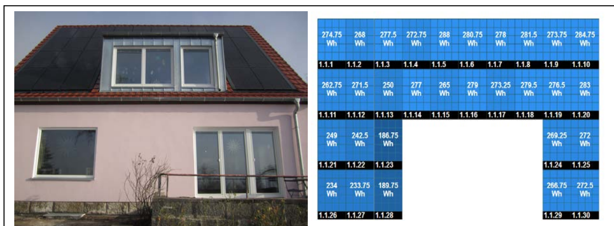
Figure 7 PV system and layout, south-west orientation (left photo of the south-west facade; right module layout with monitoring figures for each module)
