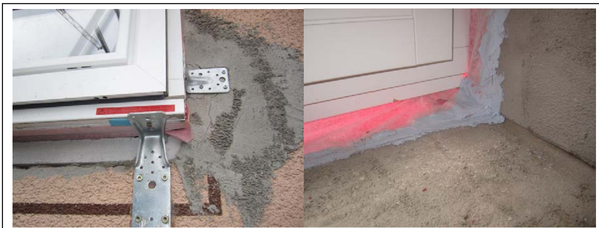
Figure 3 Left photo: construction detail of fixing the frame on to the wall; right photo: airtightness foil glued to the wall
