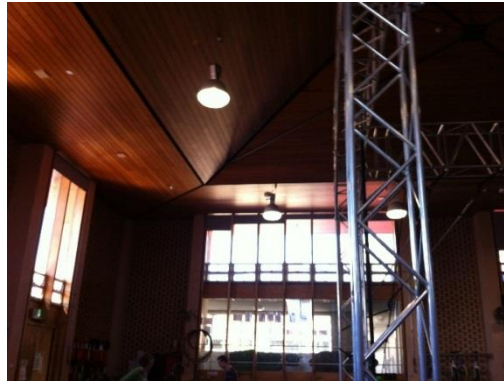
Figure 10: 250W metal halide high bays in circus hall
