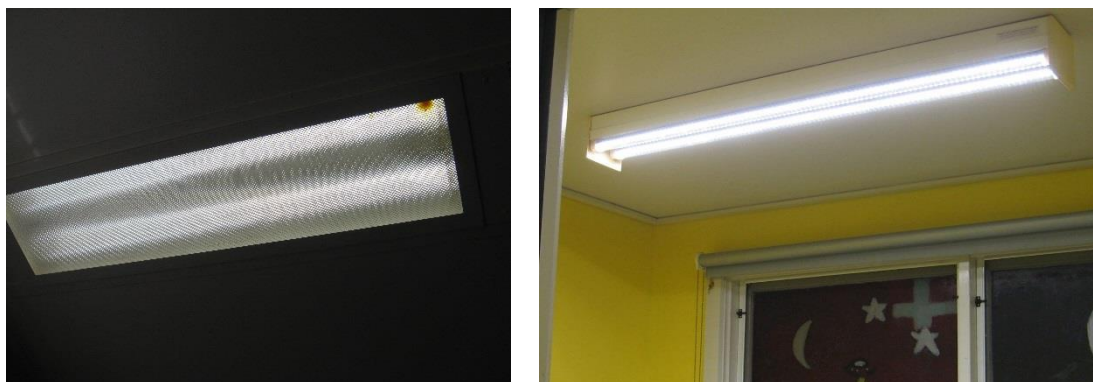
Figure 4: Reduction in glare from clear LED tubes behind fluorescent diffuser (left) versus exposed bare tubes (right)
