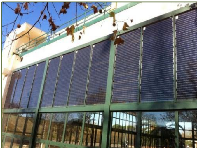
Fig. 7: CUS- Facade integrated PV glass , source [17]
