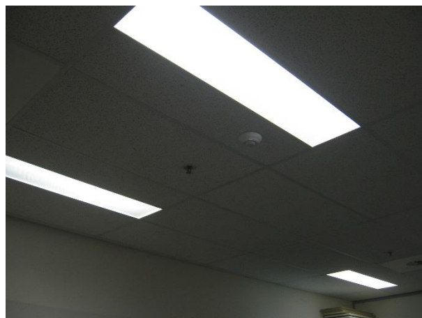
Figure 3 1x36W T8 cool white recessed troffer at Griffin Centre after upgrade
