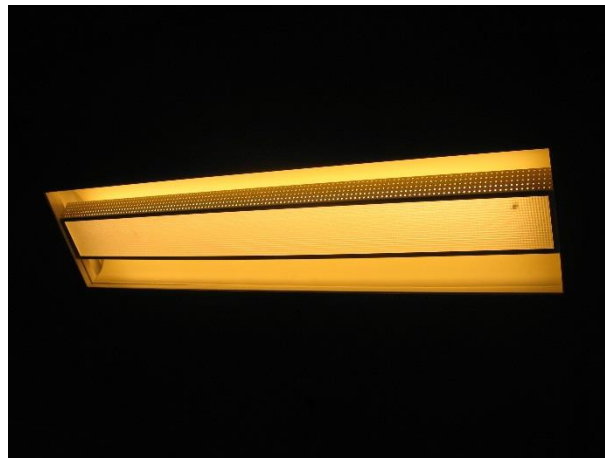
Figure 2: Original 2x36W T8 warm white recessed troffer at Griffin Centre
